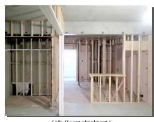
(造作工事完了)
